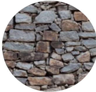
STONE MASONRY WALL
